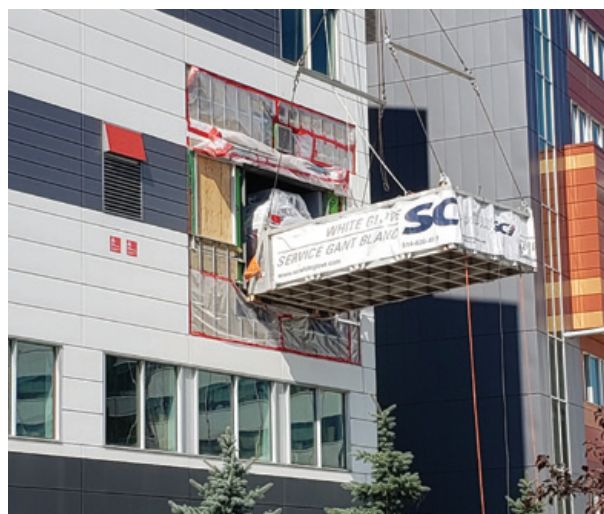
Delivery of cutting-edge cardiac MRI machine to Glen site
